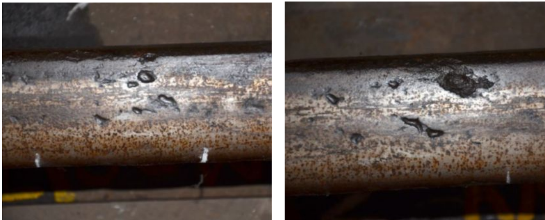
Figure 5. Sample prepared for NDT examination Rail head surfaces showing defects.
