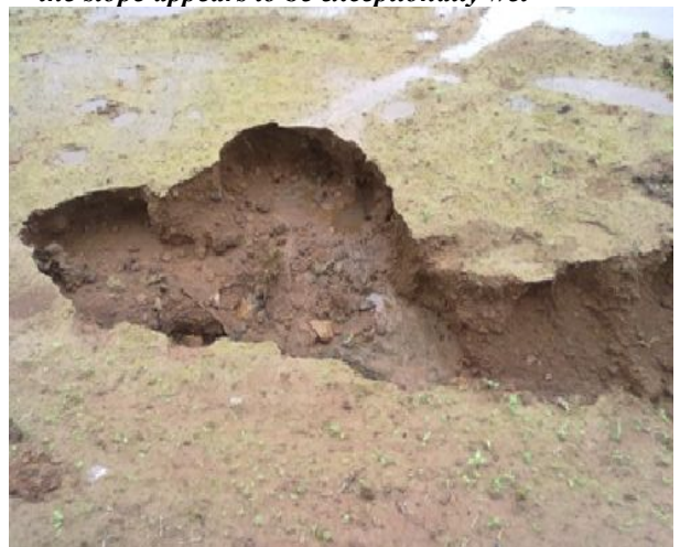
Figure No 3 : Deep rill formed due to heavy rain
